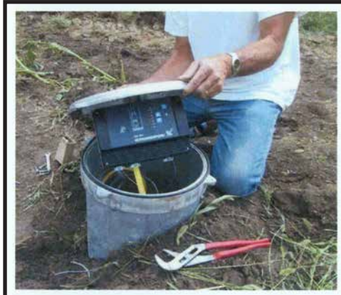
Controls mounted on plate attached to lid
